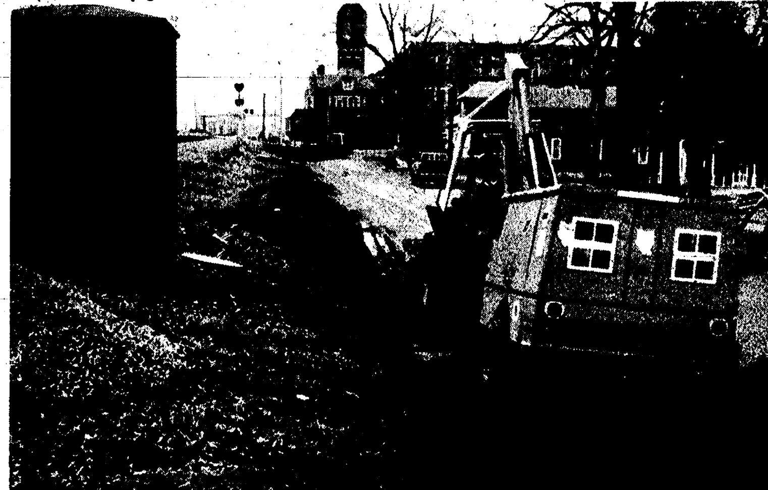
A NEW NATURAL GAS LINE is being installed along Railroad St. between East St. and McKinley St. According to company workers, a company survey crew discovered
